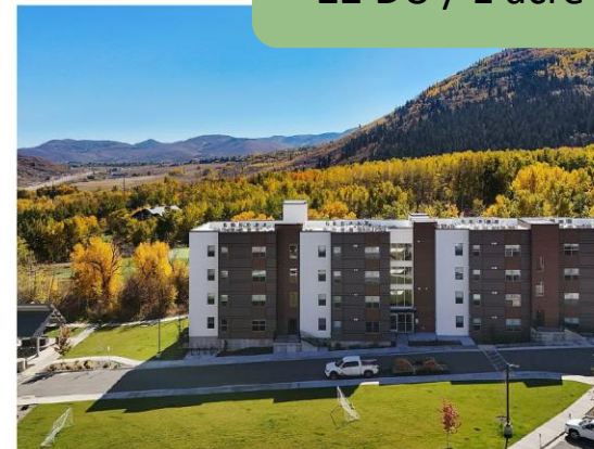
Apartment Complex – 4 stories (Park City, UT)
